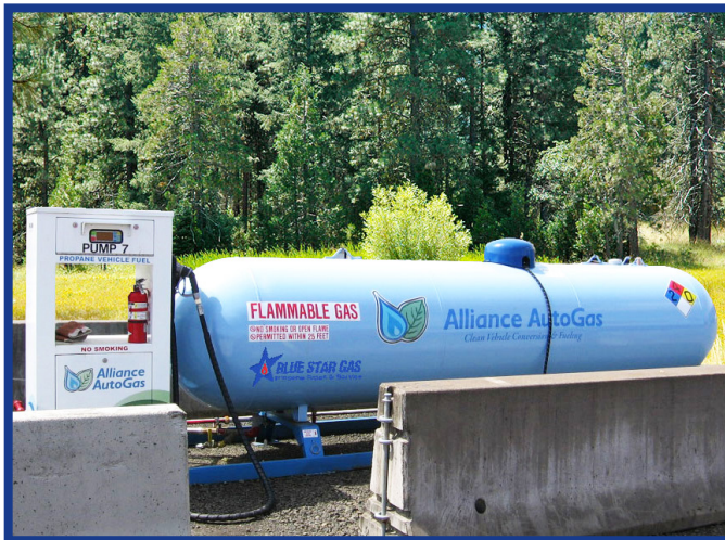
Polk County Sheriff's Office on-site fueling infrastructure
